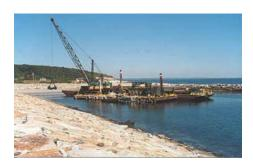
The Pilgrim Nuclear Power Plant Dredging project (40,000 cubic yards) in Plymouth, MA required precision dredging at the plant's cooling water intake structure. The turbidity controls were very stringent, due to concerns with plant turbines. Cashman employed turbidity-removal techniques successfully developed on past projects.
