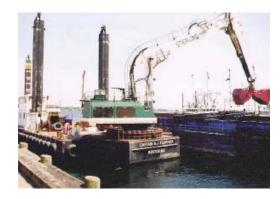
Dredged contaminated sediment alongside a pier/bulkhead at an active northeast marine facility. Material was dredged, dewatered, stabilized and disposed of at onsite upland disposal site.
