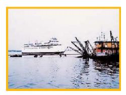
Mechanical dredging with open sea disposal performed for NE District ACOE during limited dredging "window." Dredging was in confined channel that was kept open for active commercial fishing operations for duration of project. The project included environmental protection of sea grass beds and shellfish by maintaining over 4,000 feet of silt curtain throughout the project.
